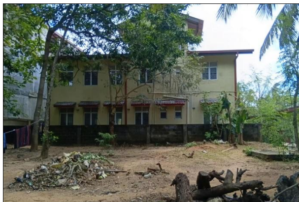
Figure 13: Government Office on Adjoining Land, Dambulla
