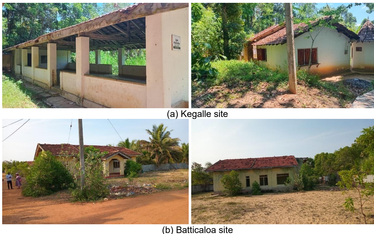
Figure C-1: Buildings to be demolished at Kegalle & Batticaloa Subproject Sites
