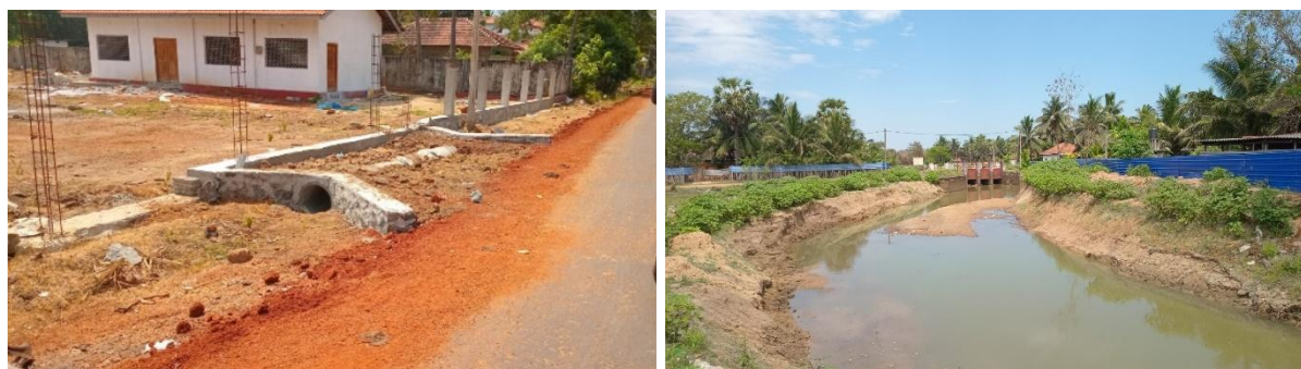
Figure B-6: Roadside drains (L) & Nay Aru irrigation system (R)
